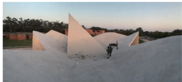
the repaired exterior roof of the Gandhi Bhawan
