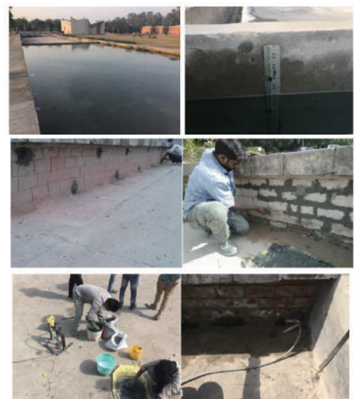
The repair process for the pool
