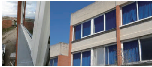
new window frame after replacement
